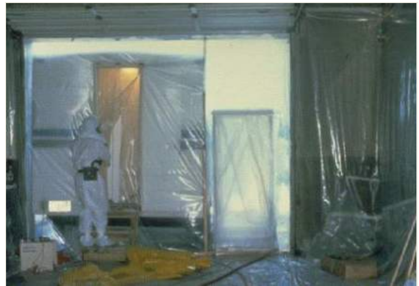
Asbestos abatement area contained and enclosed
