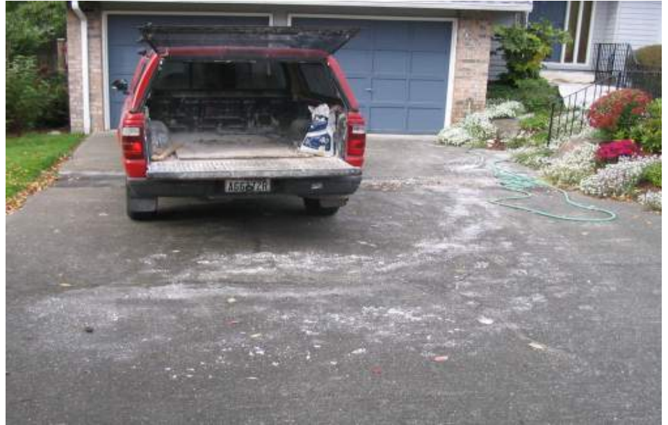
Uncontrolled popcorn ceiling removal job
