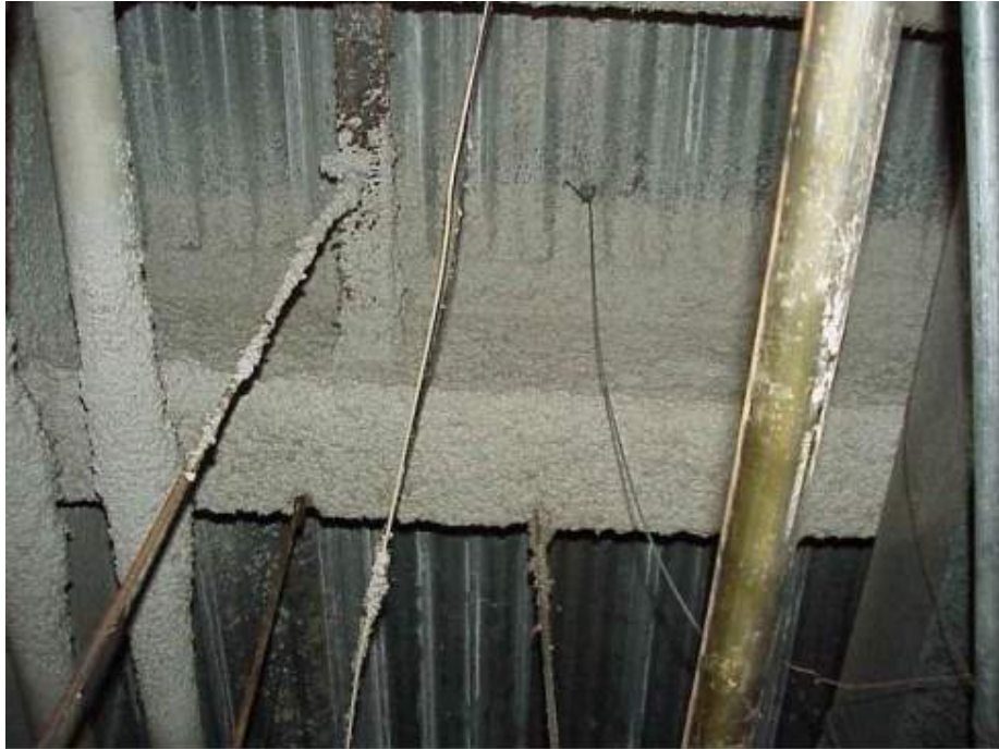
Sprayed-on fireproofing material
