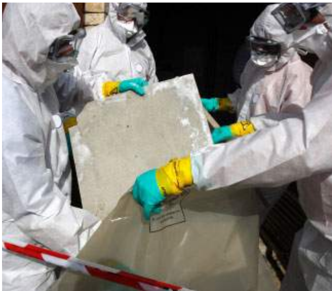
Removal done correctly
