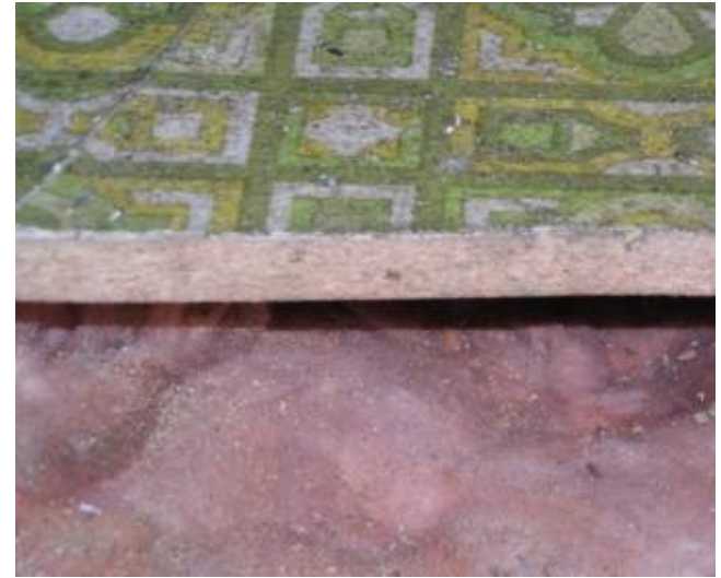
Sheet vinyl containing asbestos
