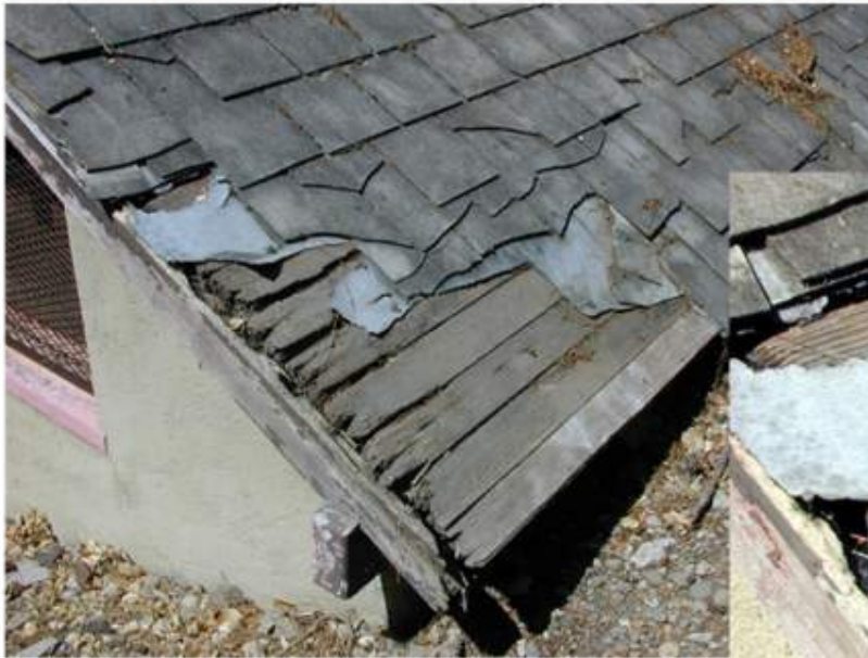
ASBESTOS CEMENT ROOF SHINGLES AND FELT (TAR PAPER)
