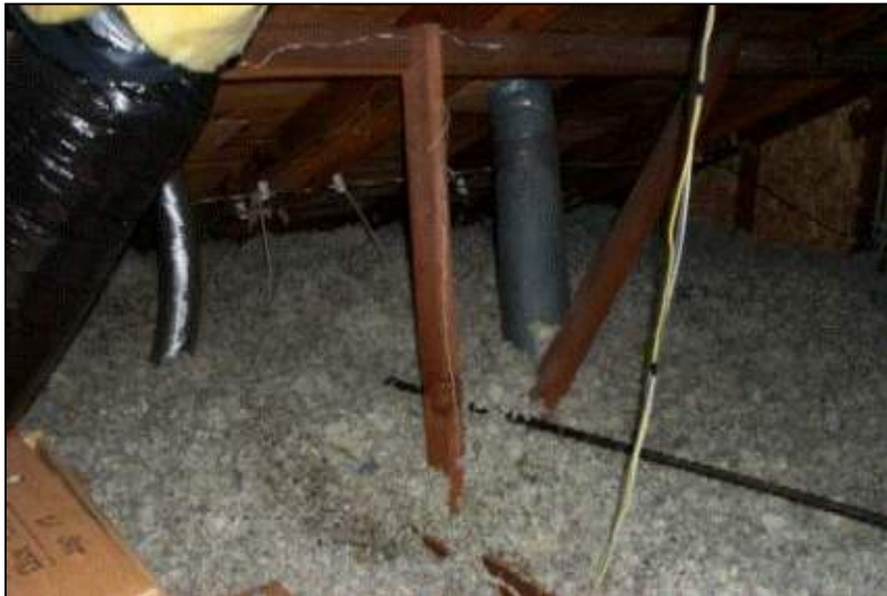
Vermiculite insulation in attics
