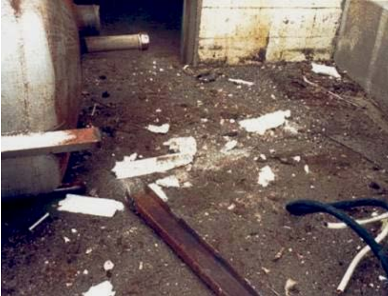
Loose asbestos debris from demolition project
